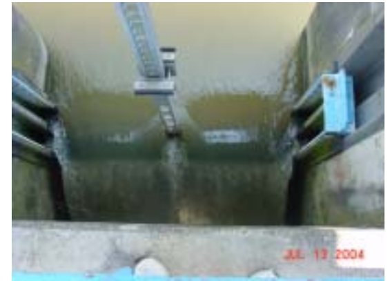
⑭-3 (県営曽根線) 笛ノ橋樋管 越流H=0.25m
