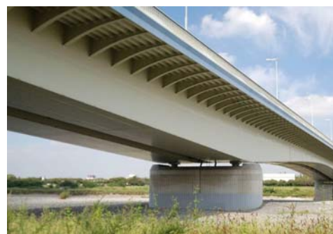
桁の溶接事例
