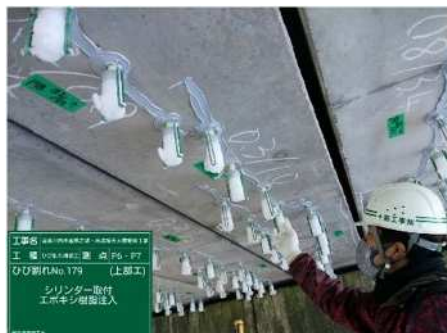
ひび割れ補修工
