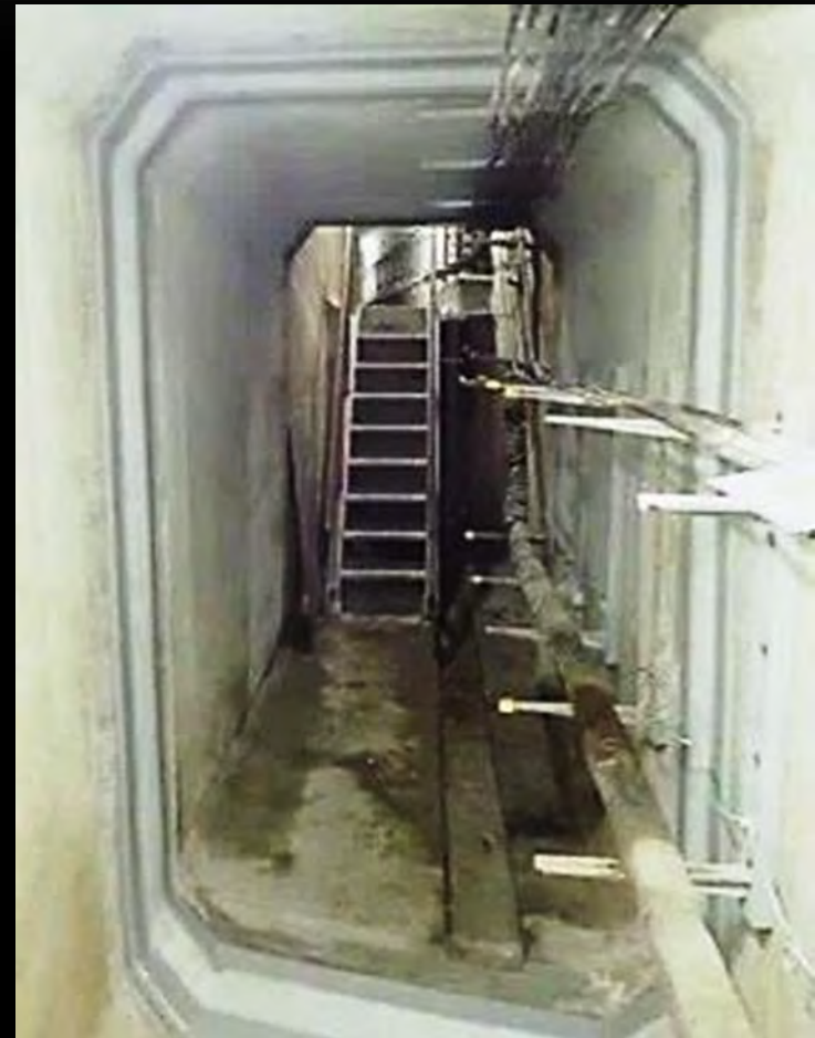
[KS工法補修後]
