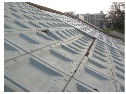
護岸の破損
