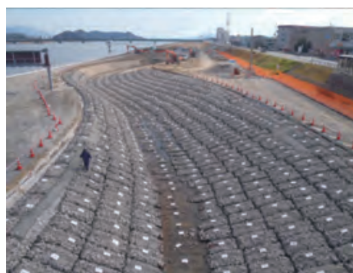
Recycled concrete pieces for underground structure. 2011. Photo: Takayuki Fukaura
