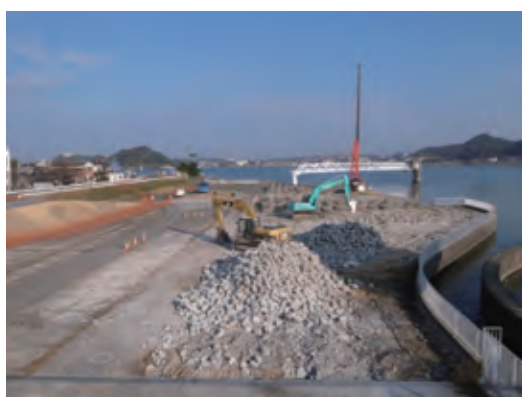
Getting rid of concrete structure, 2010. Photo: Keitaro ITO
