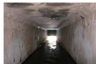
函体補修施工前
