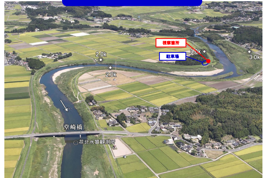
巡視②:羽月川右岸2k600付近
