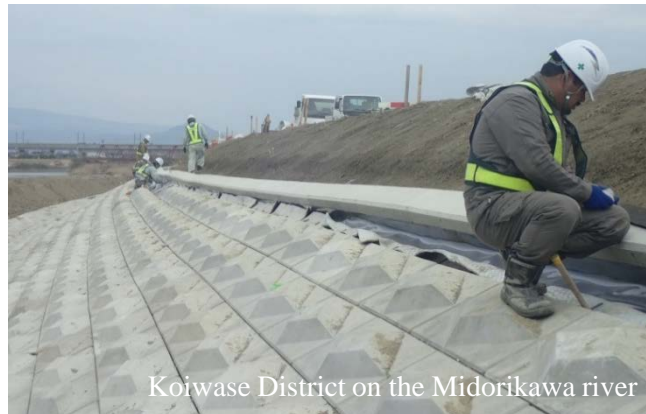
Investigation of river embankment damage
