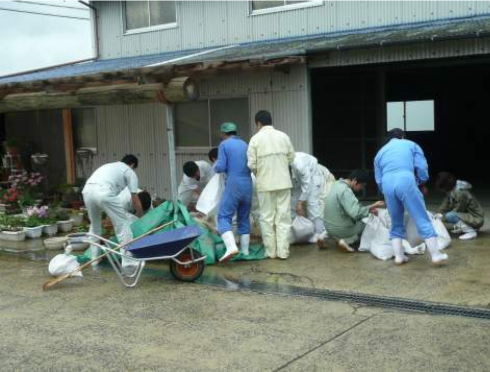
○ Placing sandbags to prevent the inundation of a barn
