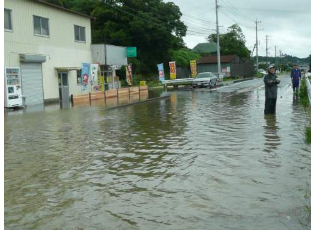
○ Placing boards to block waves
