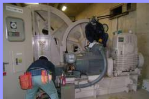
Connecting the operation panel of the conduit gate
