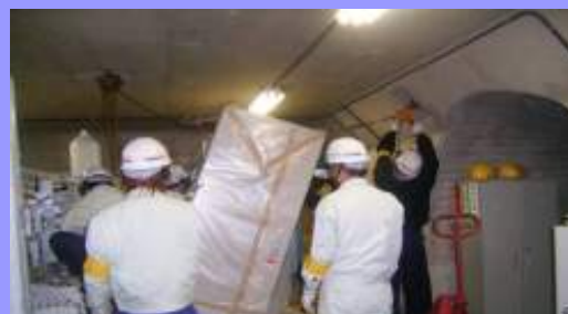
Installing the operation panel of the conduit gate
