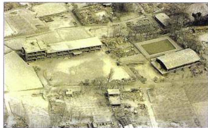
Photo.5 Ohno-Koba elementary school damaged by pyroclastic flows occurred on September 15, 1991
