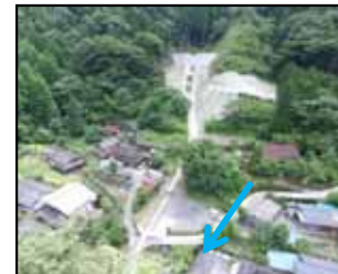
①宮園砂防堰堤 (H29.6)
