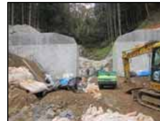
④築切砂防堰堤
