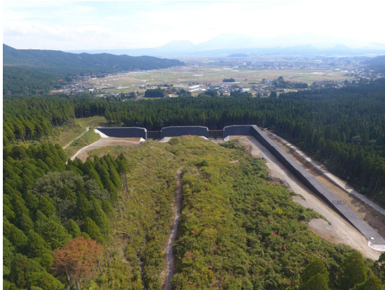
図-4 西湯浦川1砂防堰堤
