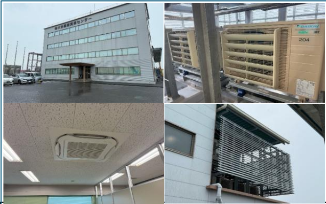
Energy Conservation in the Administration Building(Air-Conditioning System)
